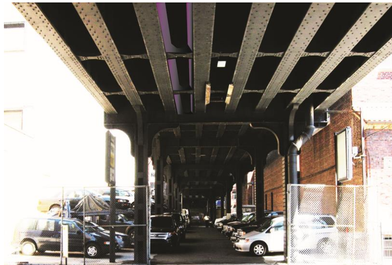
Figure 6. Rendering of Pneumatic Tube Running Between Girders on the Underside of the High Line (between the 3 rd and 4 th girders from the left) (ClosedLoops LLC, 2014)
